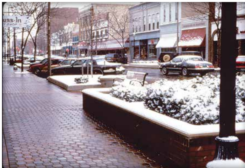
Figure 1. A snow melting system under concrete pavers in downtown Holland, Michigan has performed well since 1988.
